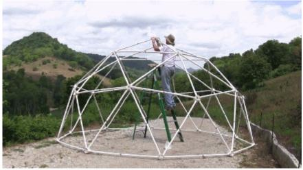
This will be a <u>tight fit</u> as the last pieces will lock the dome together. You may have to stand near the top of the ladder to apply force.
