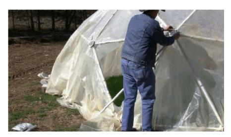
Take the second strut, and attach it in the same way to the hub at the bottom of the opening.
