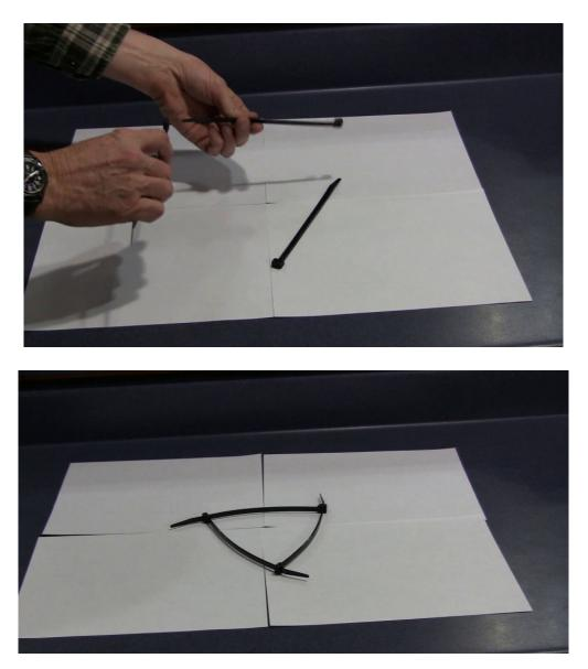
Attach the plastic to the dome by wrapping the plastic over the hub, and secure the plastic by cinching the 3 Zip Ties down over the plastic on the hub between the edge of the struts and the ridge on the outside of the hub.
