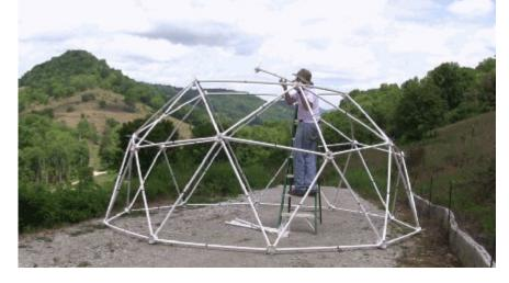
Insert the other 4 Red Struts into the hubs on the Second Tier.
