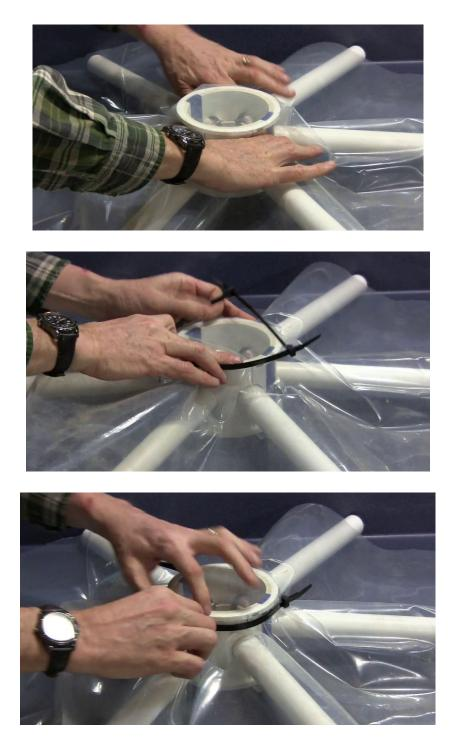
It is easier to attach two layers to the dome if you start with the covering on the inside of the dome. To do this, you will need to find the exact center of your covering material, so that it can be attached to the center, or top, of the inside of the dome.
