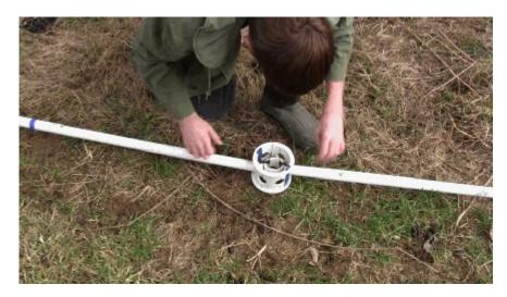
Page 6 of 35 Zip Tie Domes 1857 Brindley Hollow Road, Buffalo Valley, TN 38548 USA www.ziptiedomes.com - Telephone: (931) 858-6892 After the Zip Tie has secured the strut to the Center Ring, move the strut to where it locks in a 36 degree angle to form the circle of the foundation ring.
