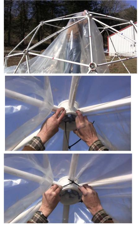
Pull the covering to the next hub, and take up any slack in the covering between the hubs. Secure the covering to all of the hubs in the interior of the dome.
