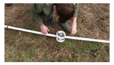
After the Zip Tie has secured the strut to the Center Ring, move the strut to where it locks in a 36 degree angle to form the circle of the foundation ring.
