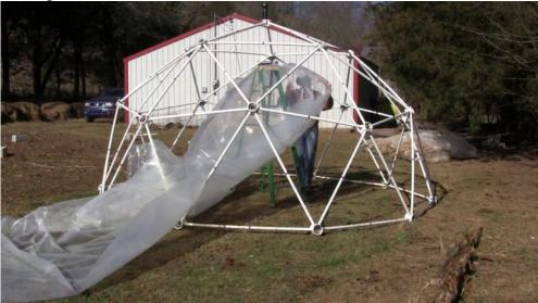
Get under the covering and place the marked center of the covering over the hub at the top of the dome. Have 3 zip ties in a daisy chain ready to cinch down the covering over the hub. You may need one or more people to help you do this.
