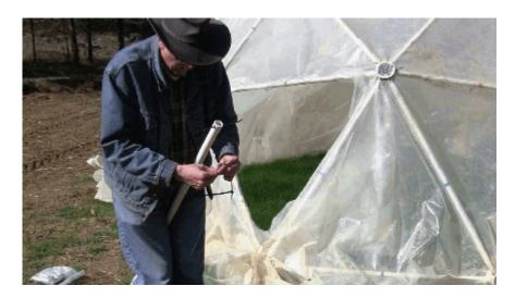
Daisy chain 3 zip ties together as shown in "How to Attach a Greenhouse Cover", and
