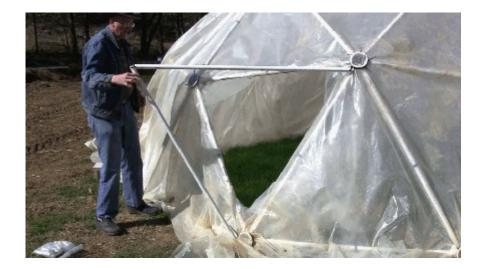
Pull the loose plastic flaps up to the door, and attach the plastic to the door with clear tape or greenhouse clips.
