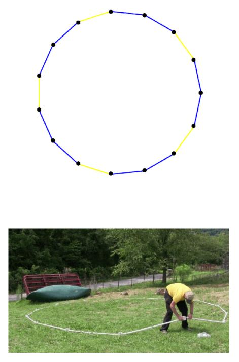
Before connecting, make sure each Hub is pointing upwards, with one of the large openings laid flat on the ground, and with the smaller openings for the struts in a horizontal position.
