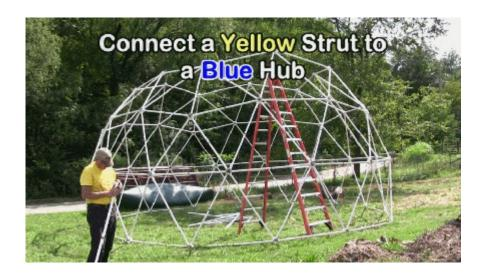
Connect 2 Blue Struts to the Hub on either side of the Yellow Strut.
