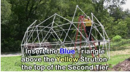
**Step 18. Connect the Top of the 3rd Tier with 10 Blue Struts.**
