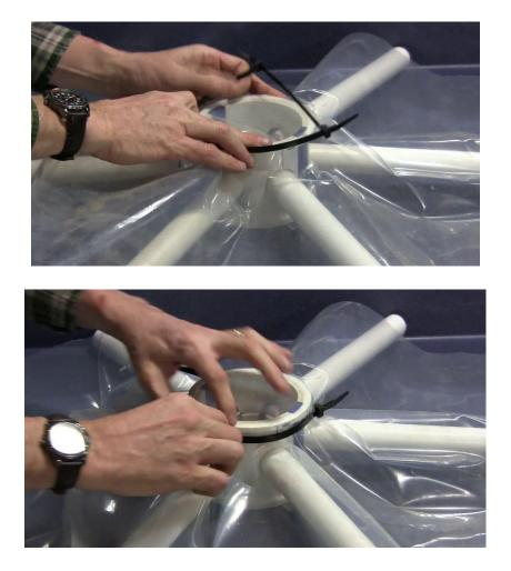
It is easier to attach two layers to the dome if you start with the covering on the inside of the dome. To do this, you will need to find the exact center of your covering material, so that it can be attached to the center, or top, of the inside of the dome.
