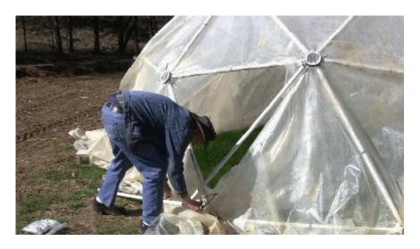
To make the door, connect the loose ends of the two struts together using two zip ties.
