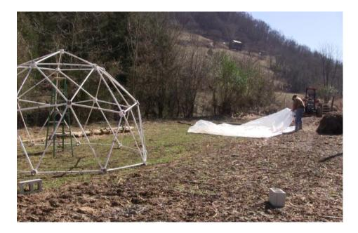
Find where the double fold is, and make a large, visible mark with an ink marker to mark the center of the covering.
