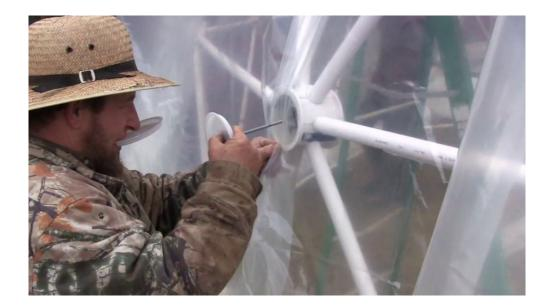
Push the Test Cap into the hub opening, securing the greenhouse covering to the hub. On the inside of the dome, thread a Test Cap over the carriage bolt, and secure with a washer and nut.
